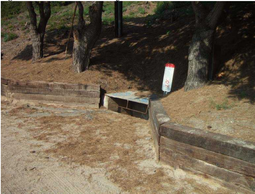
Figure 2-9. Treated wood retaining wall
